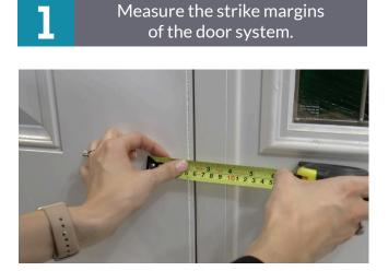
**a.** Measure the space between your door panel and door frame where the strike plates are installed.
