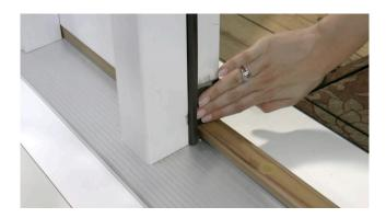
**a.** Once you have both the vertical and horizontal alignment set, press the corner pad firmly against the jamb.
