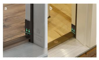
**a.** If you have an Endura Z-Articulating Cap Sill<sup>™</sup>, align the corner pad flush against the Z-End Base<sup>™</sup>, or the black stiffener.
