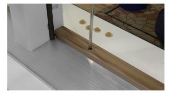
a. Tighten or loosen each adjustment screw a small amount to achieve the desired height.
