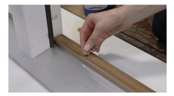
**a.** Place the cap plug over the cap hole and press down firmly. You may use a rubber mallet to secure the plugs.
